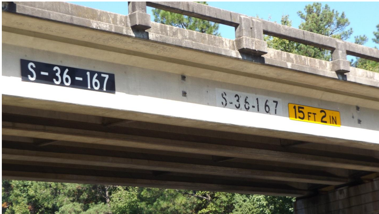
Figure 10 - Vertical Clearance
