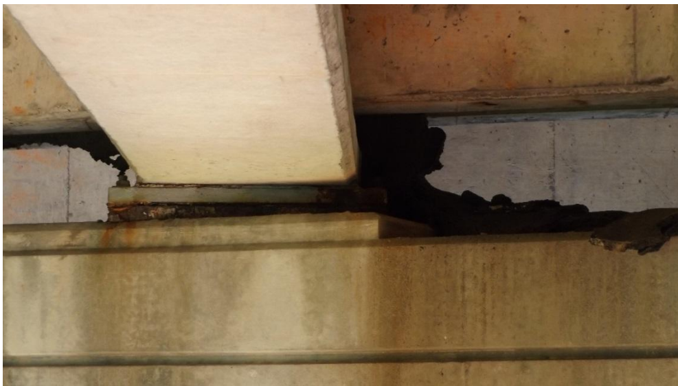
Figure 7 - Expansion Joint material falling through joint opening
