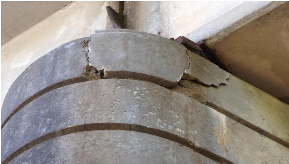
Figure 9 - Spall on Top of Pier Cap
