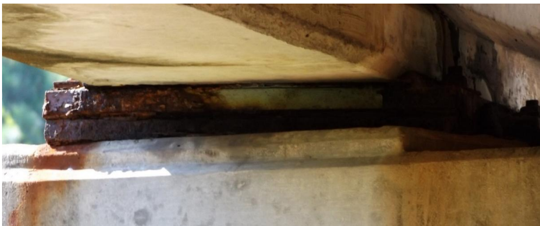
Figure 5 - Bearing Corrosion
